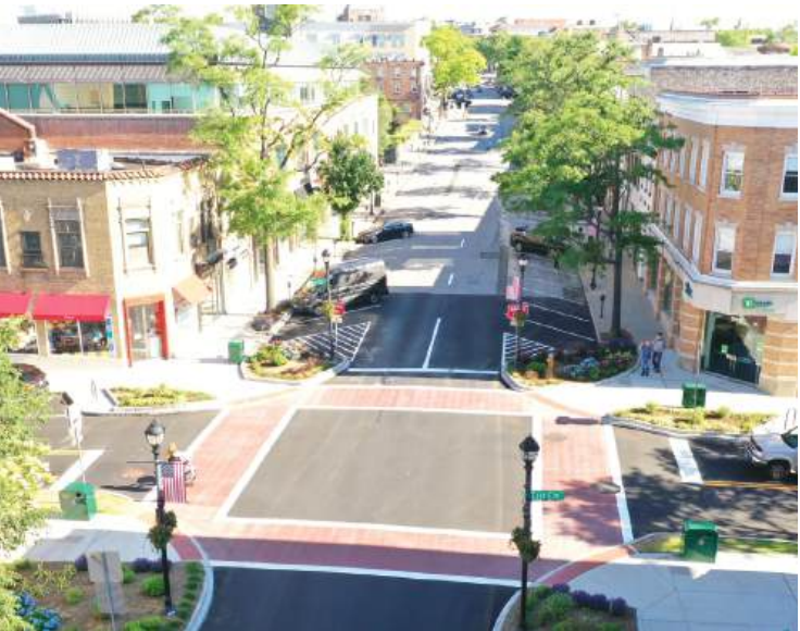
4d Vehicle parking which compliments pedestrian movement
