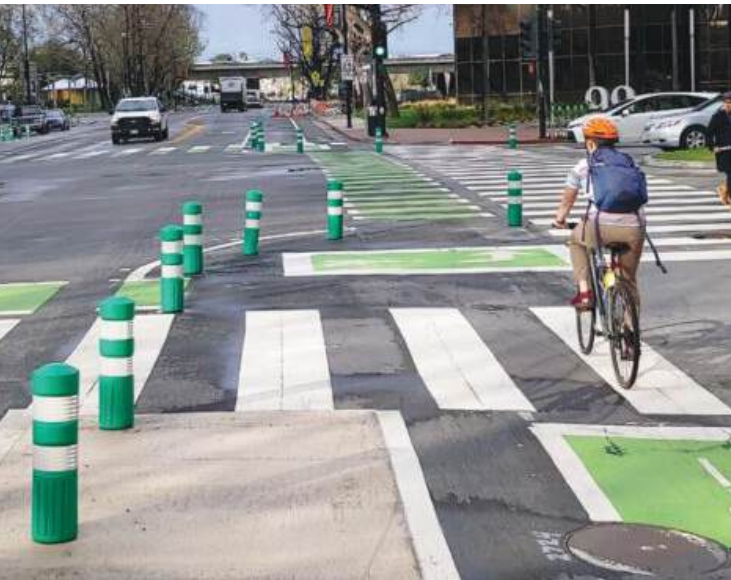
4b Infrastructure improvements to improve safety
