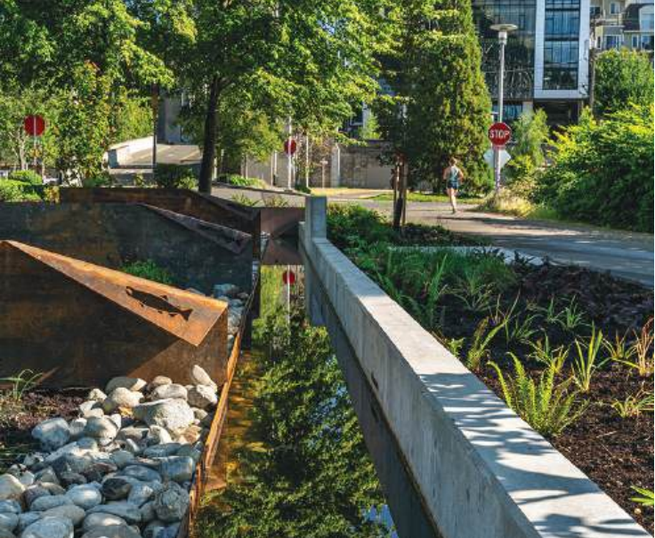
8c Stormwater infrastructure
