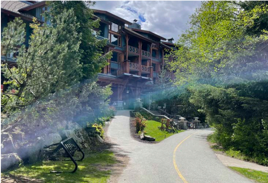
Figure 12: Valley Trail and bike storage along Nita Lake.
