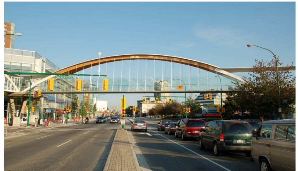
Figure 23: Kingsway Pedestrian Bridge, Burnaby. Image courtesy of Fast+Epp.
